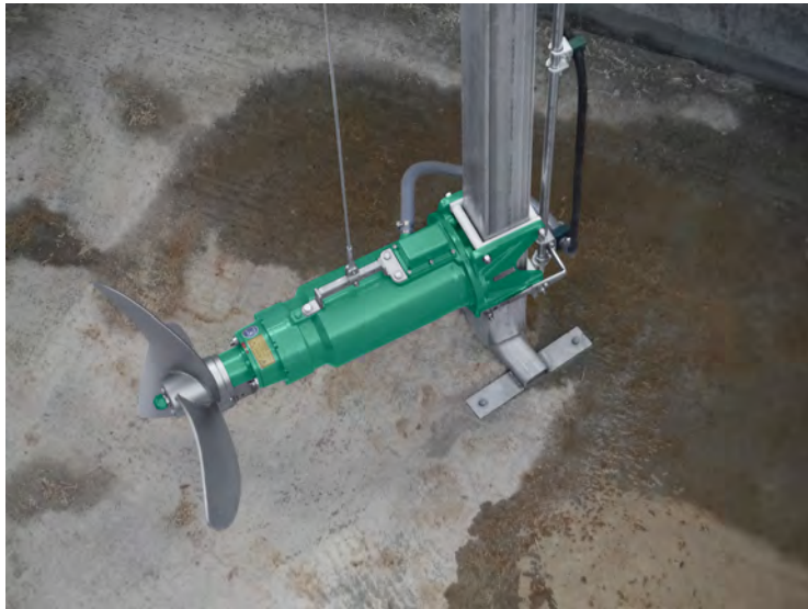
3G - Concrete tank
